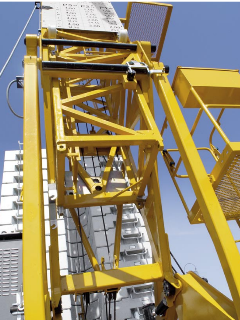
Further tower sections are inserted for greater hook heights.
